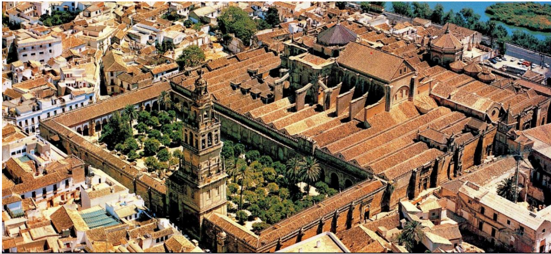
Image no. 9: Aerial view of the courtyard of the Great Mosque of Cordoba, Spain. (Sanguedolce, 2008). The space which is covered with trees is a courtyard inside the mosque.
