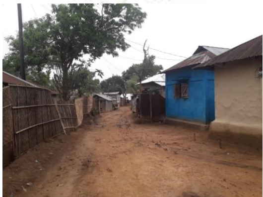
Figure 3.1.33 Mud and Brick Houses along Mud road
