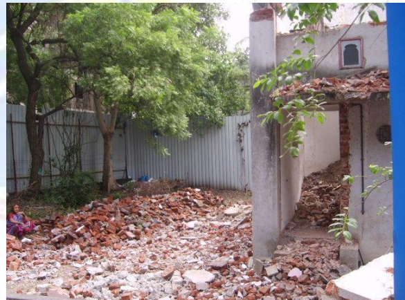
Fig. 4- Bricks cleaned off mortar and sold to slum dwellers
