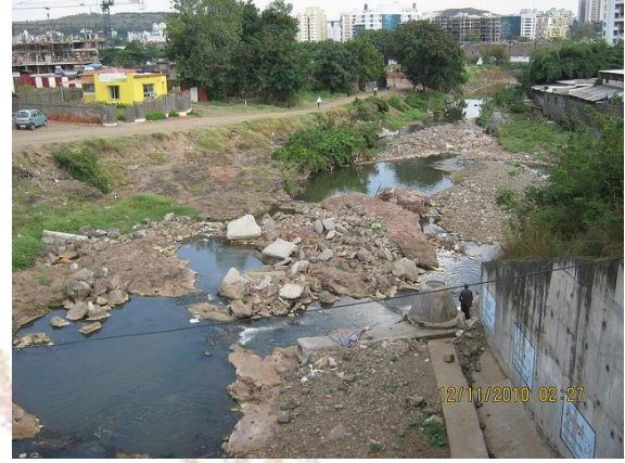
Fig.2- Dumping of debris into river bed has resulted into reduction of river width of RamnadiTNN reports
