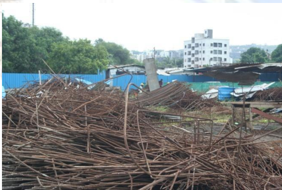
Fig. 3- Segregation at source, reinforcing steel
