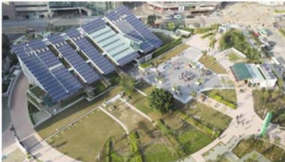
Onsite installed Solar PV Panels
