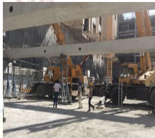
Figure 7: Assembly of a joined beam
