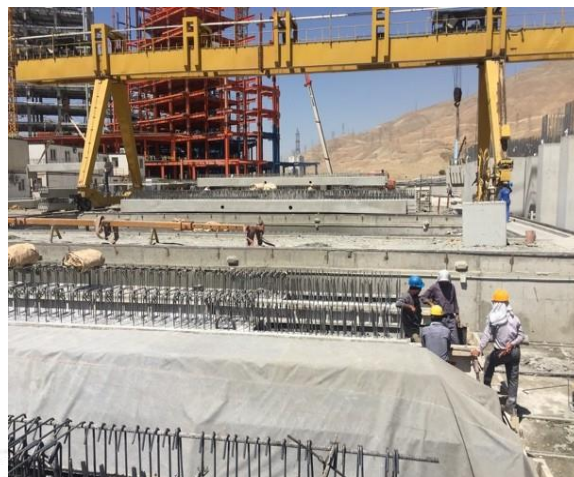
Figure 5: Curing process of concrete beams
