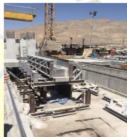
Figure 6: Column production line (Source- Time comparison between precast and conventional construction)
