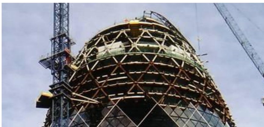
Fig 9 (b): Facade construction of the 30 St. Mary Axe
