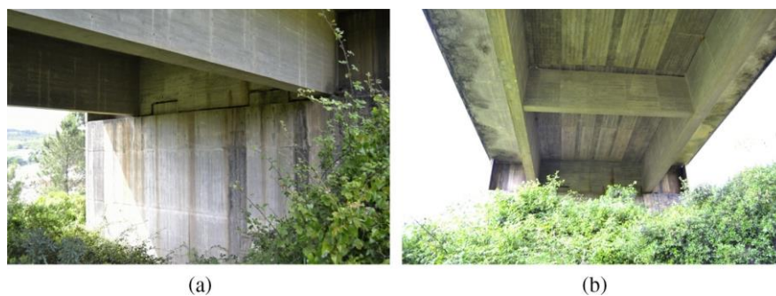
Fig. 15. Details of the north abutment: (a) East view; (b) bottom view.
