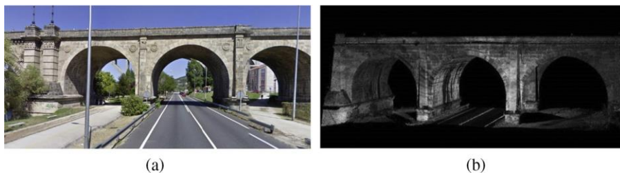
Fig. 3. New Bridge of Ourense, Spain: (a) overview; (b) 3D geometric model (point cloud) obtained by laser scanning.
