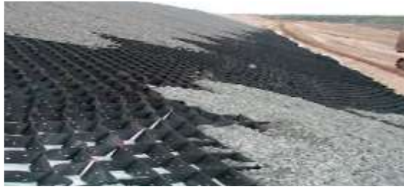
Fig.2. Reinforcement of the slope with three-dimensional geogrids
